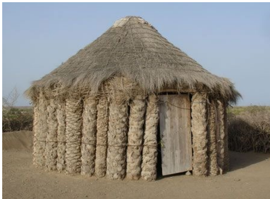
Fig. 13. Typical Tihama house, Palm trunk construction and thatched roof, Yemen, https://www.pinterest.com/artebitarealb/ (accessed September 28, 2023)
